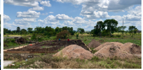
First stage of Construction of the Early Childhood Intervention Centre
