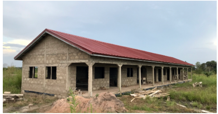
Construction of the Early Childhood Centre
